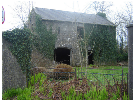
Photo 10i: Two storey cut stone building with fine arches
