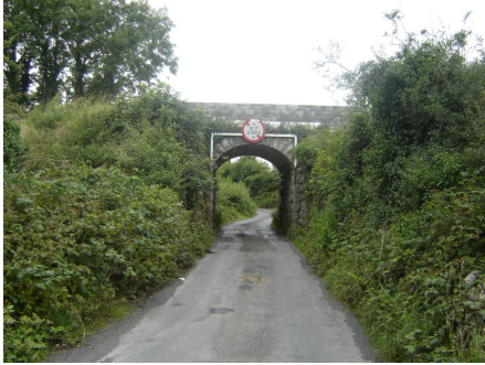
Photo 10l: Railway Bridge over local road L-3113-0
