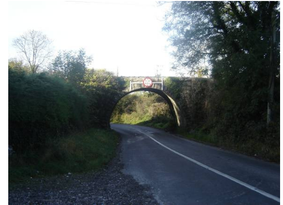
Photo 3i: Railway Bridge, Ardrahan Road (R347)
