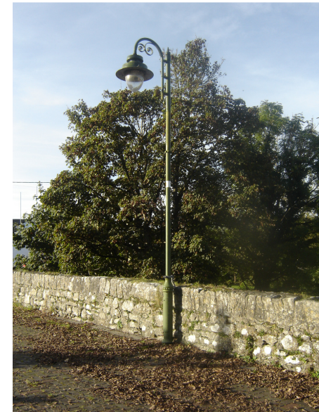
Photo 8a: Street Light on Craughwell Bridge
