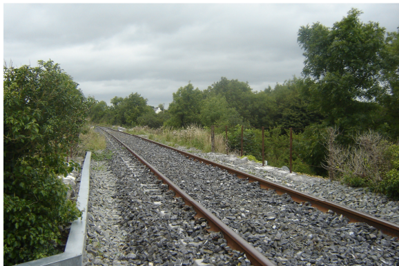
Photo 3j: Railway Track over Ardrahan Road Bridge
